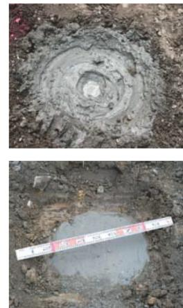
This method make high strength improvement cement column into the ground by the especially equipment. Even if bearing layer is deep, the effect is obtained. The soil can be improved low vibration, low environmental pollution, and low cost.
